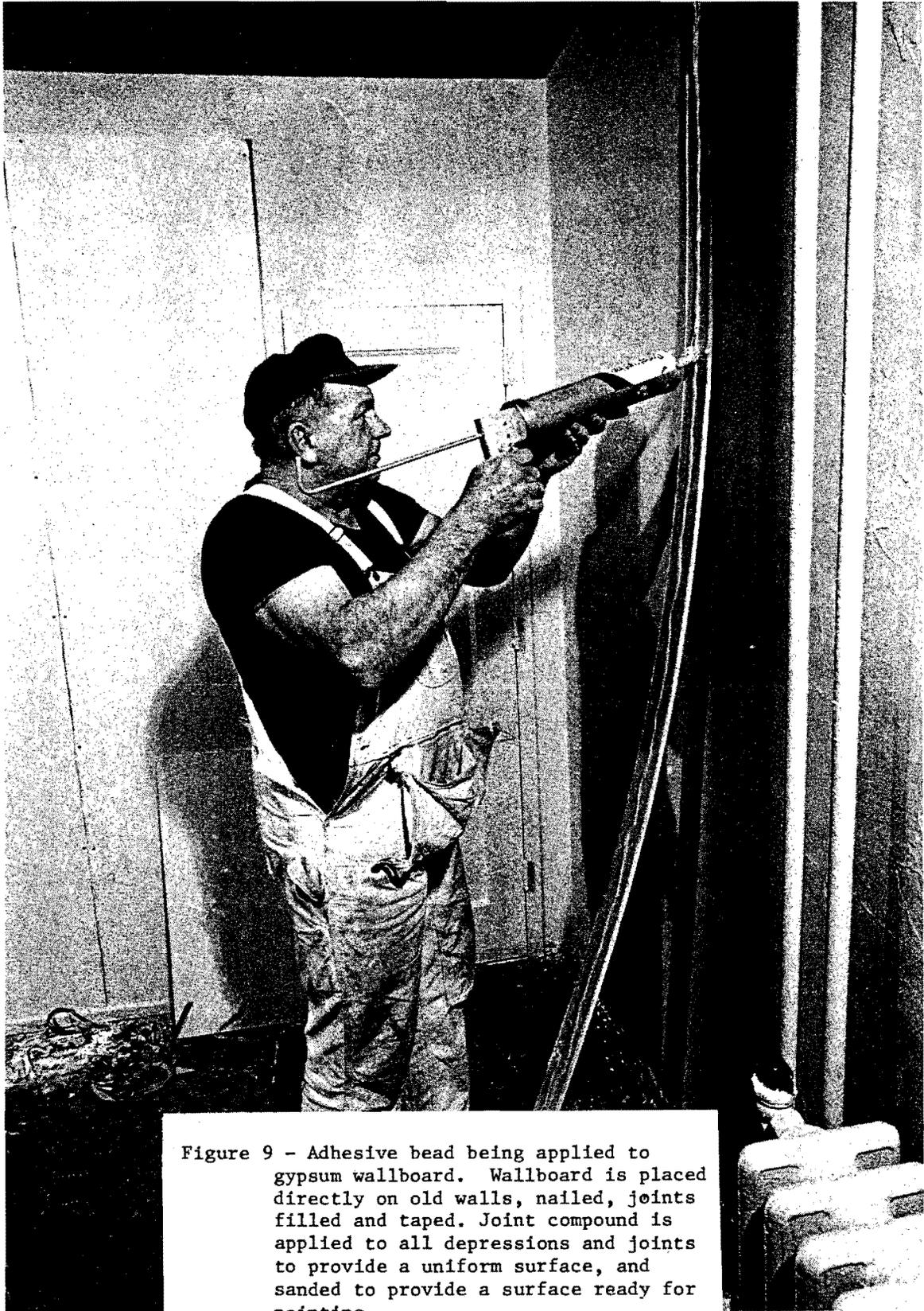
Figure 9 - Adhesive bead being applied to gypsum wallboard. Wallboard is placed directly on old walls, nailed, joints filled and taped. Joint compound is applied to all depressions and joints to provide a uniform surface, and sanded to provide a surface ready for painting.
