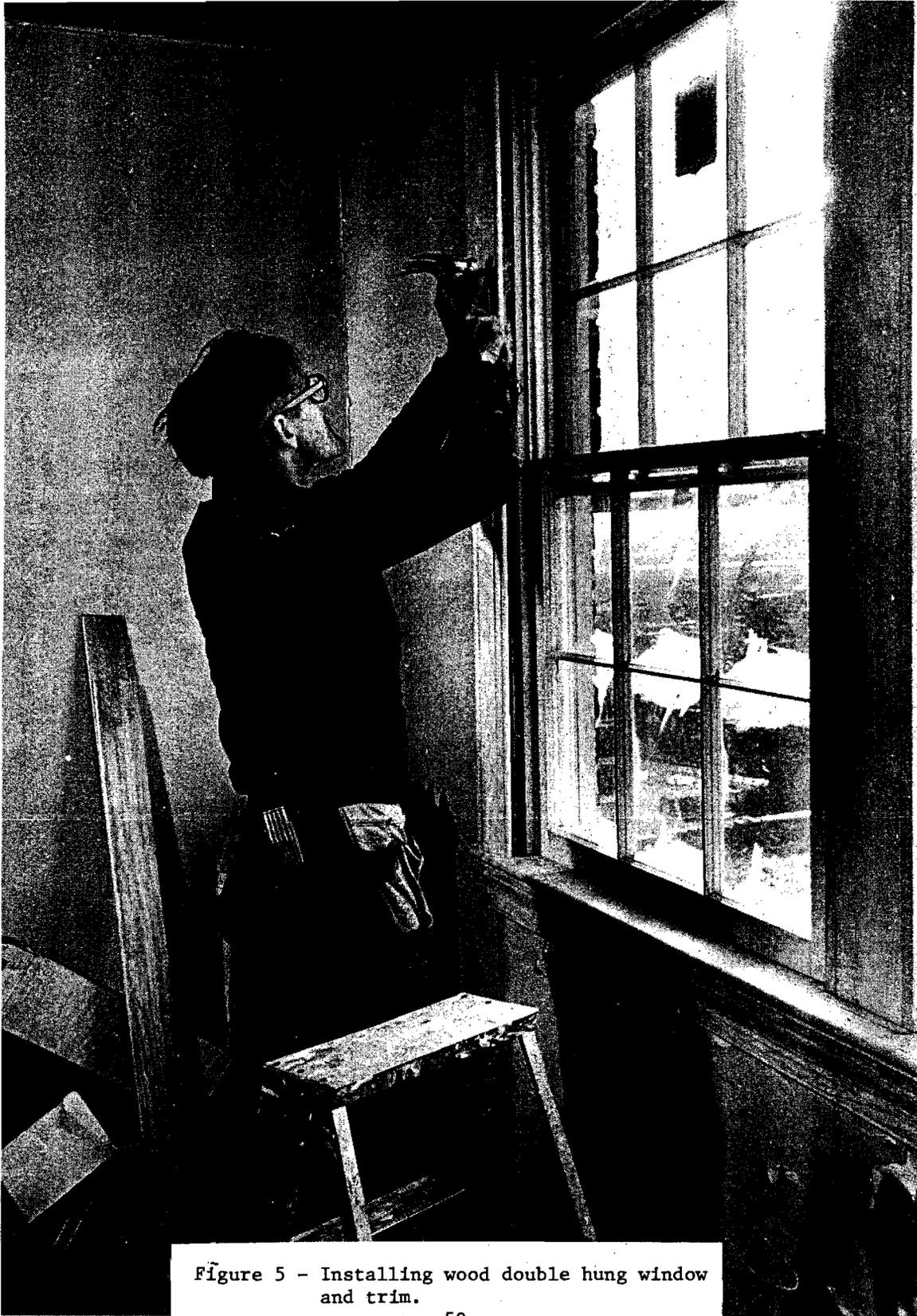
Figure 5 - Installing wood double hung window and trim.
