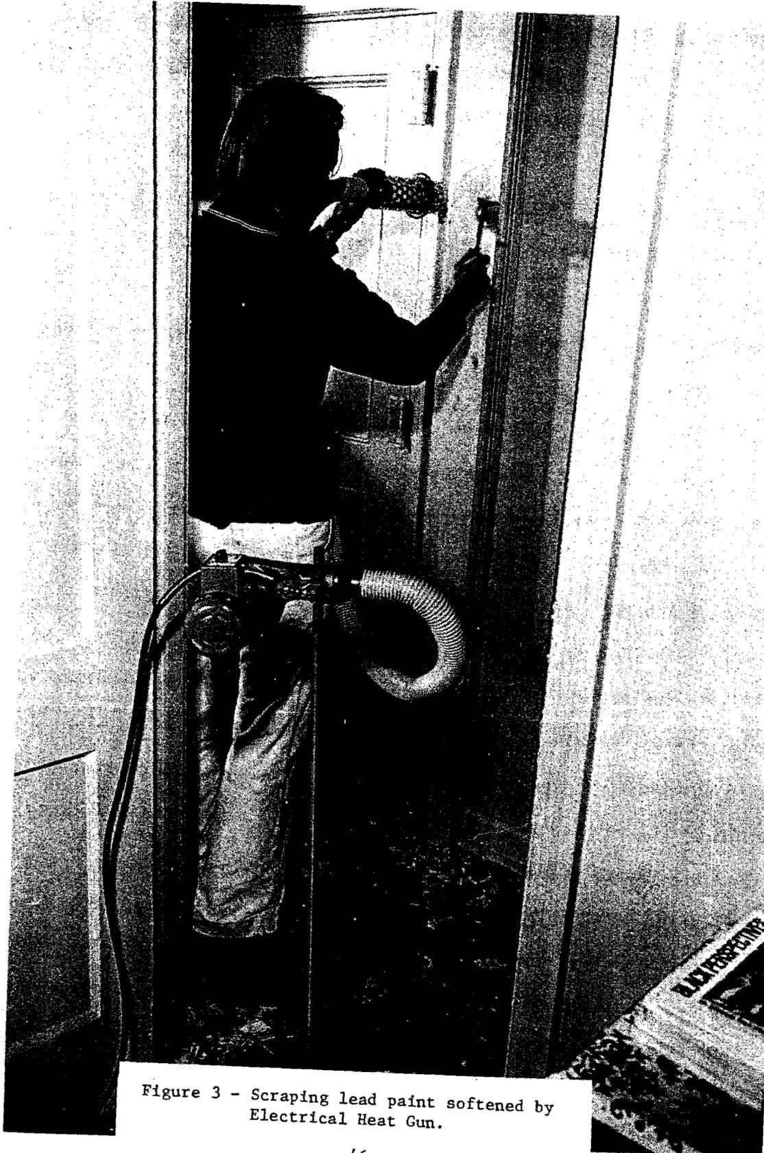
Figure 3 - Scraping lead paint softened by
